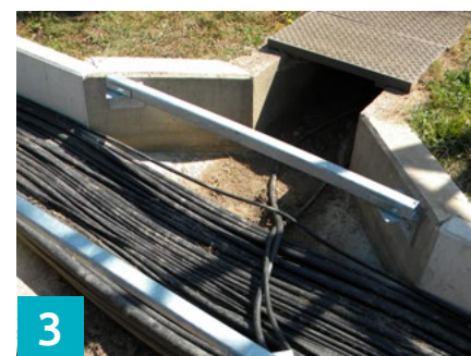
3 Fitting the square tube (50 × 50 mm) into the angle bracket.
