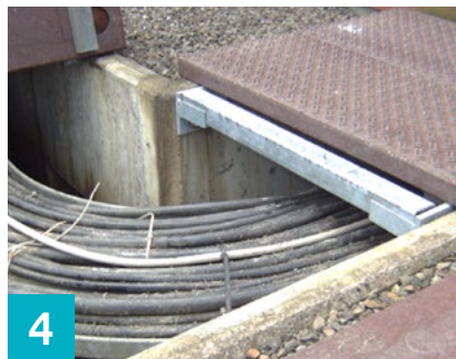
4 Fitting the square tube (50 × 50 mm) into the angle brackets.
