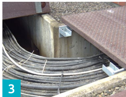
3 Fasten the two 90° angle shoes with two M10 bolt anchors per angle bracket.
