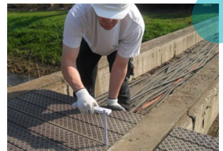
Our tip: use a folding rule as a spacer.
