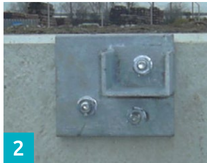
2 Use of prefabricated 90° angle brackets.
